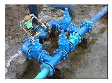
This example uses a 50mm BERMAD model WD-923 hydrometer with low flow bypass on a 90mm HPPE water main. Install cost was approximately 6000 Euros. Install time is approximately 1 week including the chamber and cover.
