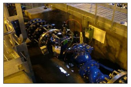
The above install took six months to construct as the chamber is 6 meters deep and the flanges and all fittings are PN25 rated. The install cost was 850,000 Euros.
